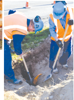
careful potholing using non-conductive hand tools
