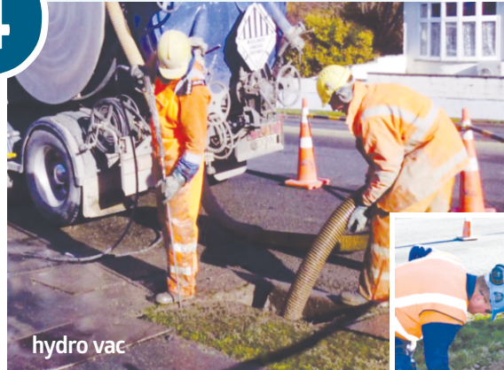
careful potholing using non-conductive hand tools
