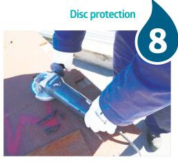
Ensure the disc has stopped spinning before placing the grinder down
